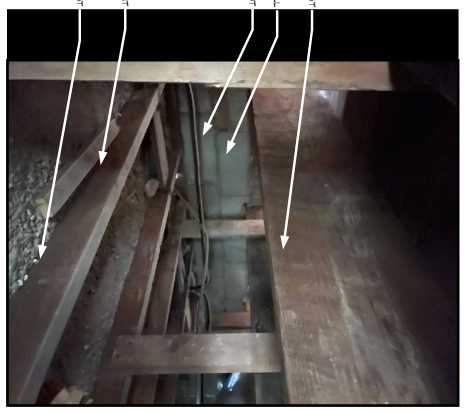
1 EXISTING CEILING SPACE AT FRONT OF BUILDING SCALE: NTS
