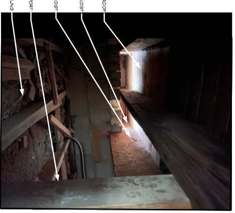
4 EXISTING CEILING SPACE AT FRONT OF BUILDING SCALE: NTS
