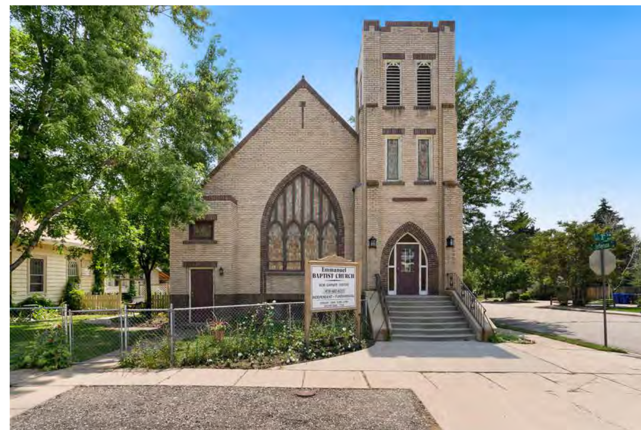
EXISTING CONDITIONS: NORTH ELEVATION
