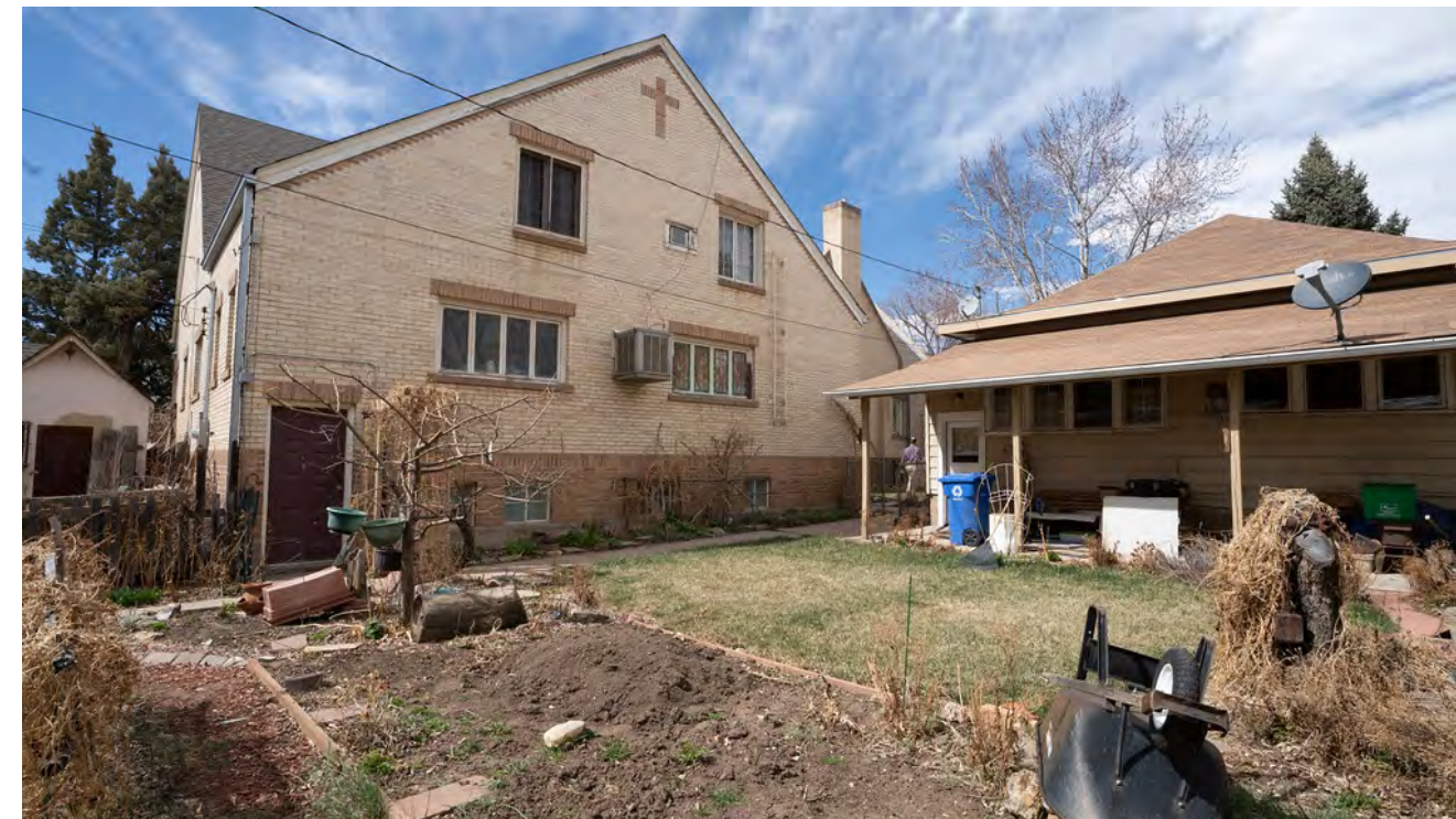
EXISTING CONDITIONS: EAST ELEVATION
